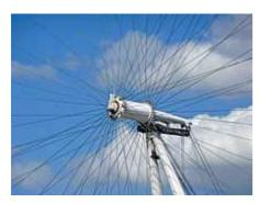
The spindle, hub, and tensioned cables that support the rim
